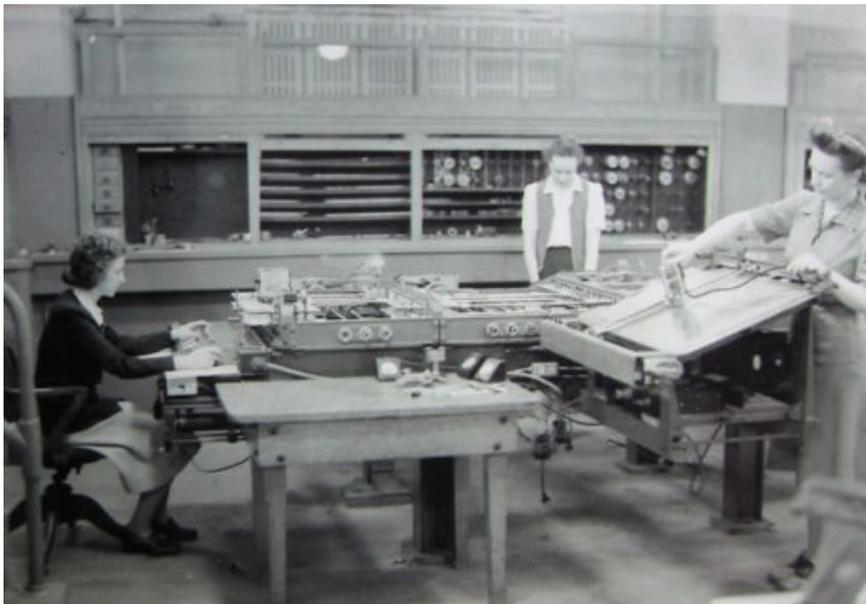
Kay McNulty, Alyse Snyder, and Sis Stump operate the differential analyser in the basement of the Moore School of Electrical Engineering, University of Pennsylvania, Philadelphia, Pennsylvania, circa 1942–1945
